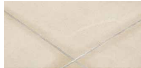
GROUTED CONCRETE PAVING
